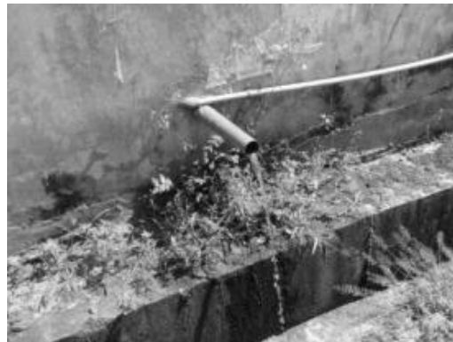
Figure 13: Grey water draining directly into the canal
